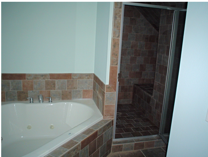
Master bath with tile shower and jetted tub
